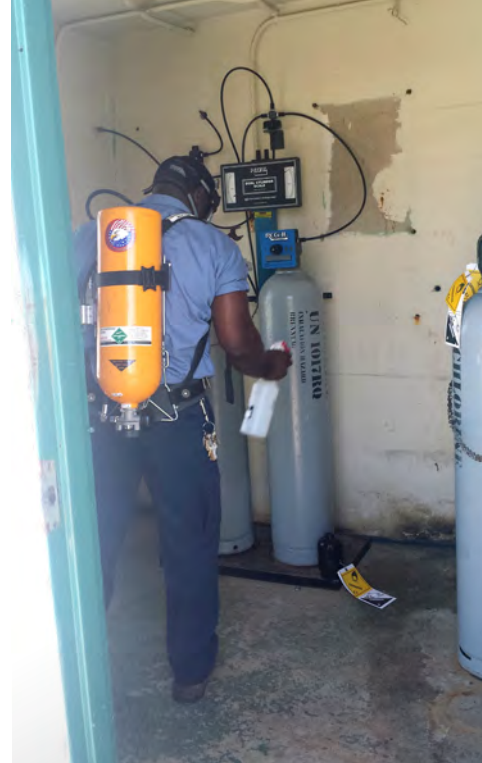
James Daniels prepares for installation of additional chlorine dosing system.
