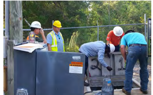
Lift Station Project City of Warner Robins, Georgia
