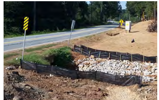
Highway 81 Water Main Replacement Project City of Winder, Georgia
