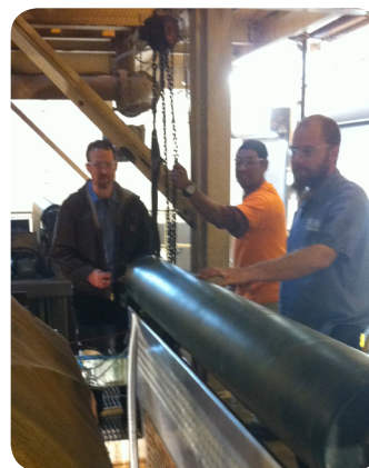
Belt Press Rehab Project
