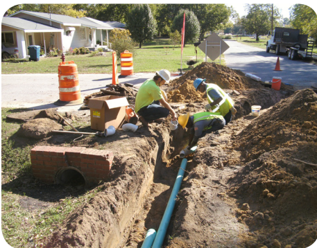
Second Street Sewer Extension Jarod Noble, Tracy Fluellen and Terry Lester
