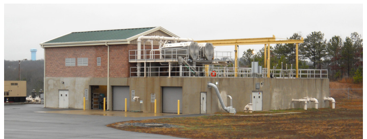
Forsyth County's James Creek WWTTP
