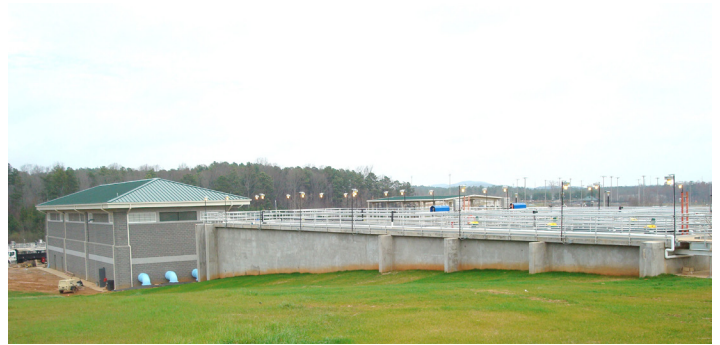
12 MGD Plant Expansion • Forsyth County
