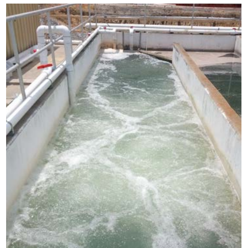
New diffusers installed in Clarifier 2 Contact Chamber
