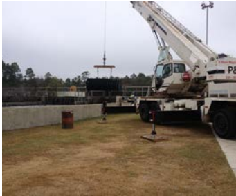
Mickey Roberts directs a crane removing an aerator section for repair
