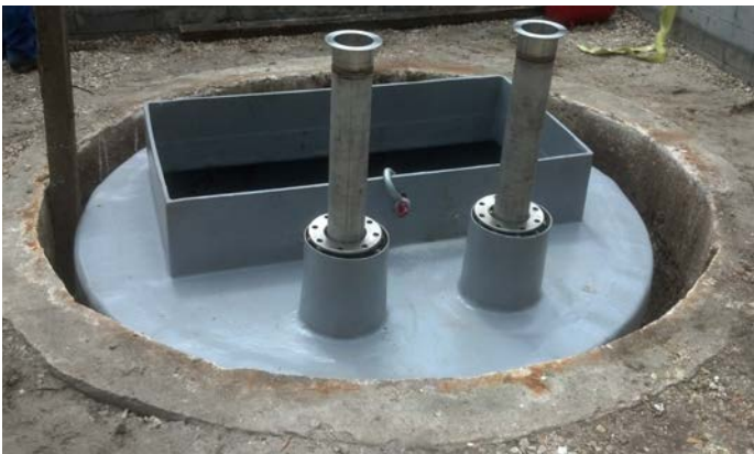
Top —NEW fiberglass wet well structure with stainless piping arrives on site Bottom —Structure set in wet well and “shimmed” to remain plumb and level
