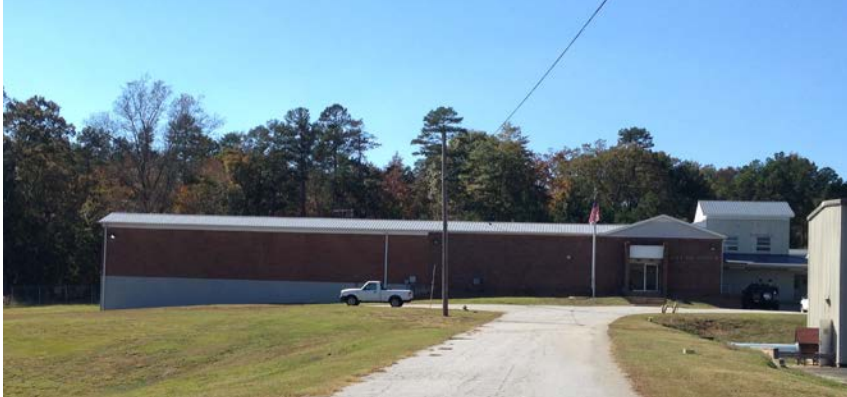
City of Winder Water Treatment Plant
