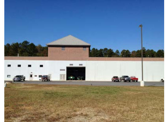
City of Winder Wastewater Treatment Plant
