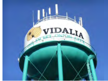
AFTER UTV RENOVATION
