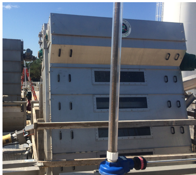
New headworks at Sandy Run
