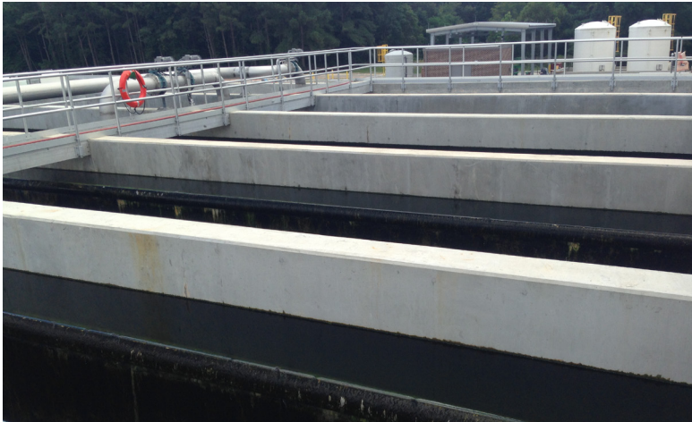
New gravity sand filters at Sandy Run WWTP
