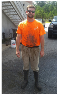
Project Manager Percy Nolan assisting with membrane cleaning
