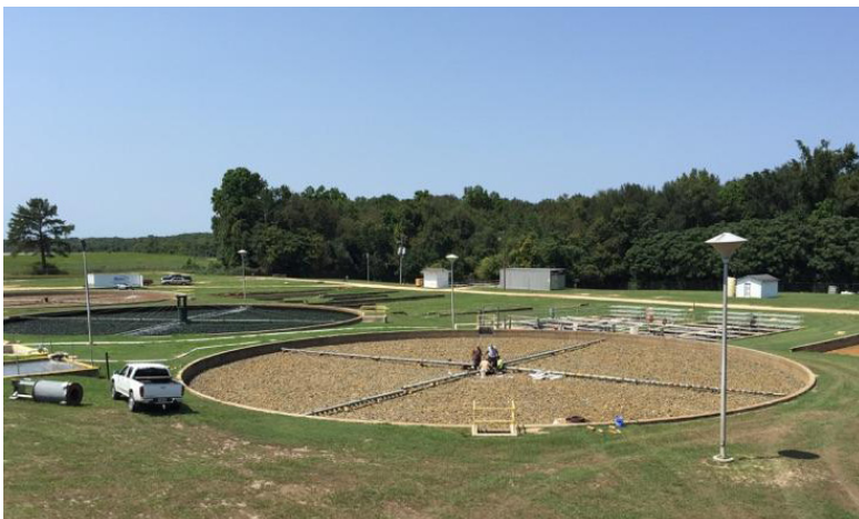
Constantine Engineering working on clarifiers at Ocmulgee WPCP
