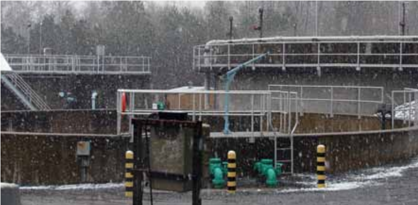
Forsyth County's Dick Creek WWTP in the snow • February 2010
