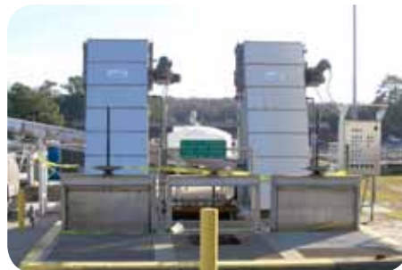
The installation of new Parkson Barscreens
