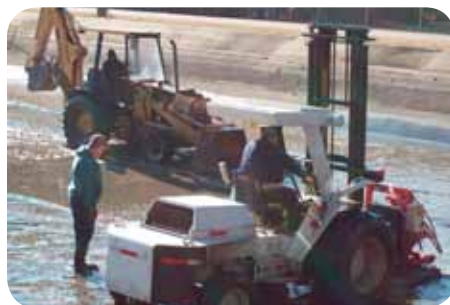
Outfall Pond Cleaning in Warner Robins
