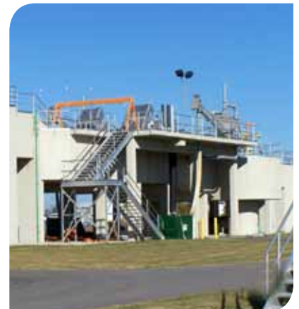
Headworks at ESG/Tupelo
