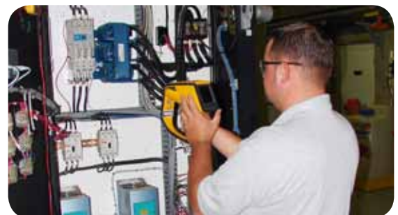
Performing in-house conditions assessment
