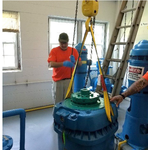
Installing Rebuilt High Service Pump Motor
