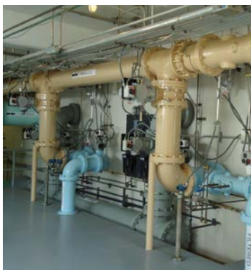
Refurbished Pipe Gallery
