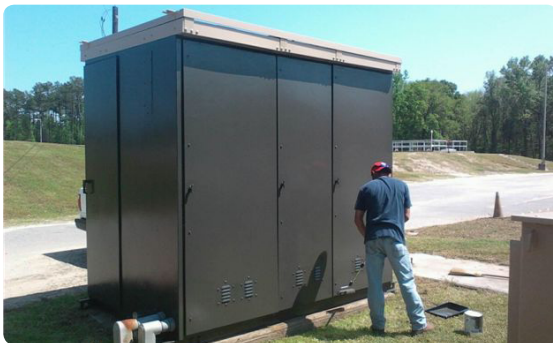
Operations personnel began “spring” cleaning throughout the WWTP. Earl Shouse (WW Operator) is shown painting the control room to match the new colors of the Operations Building.
