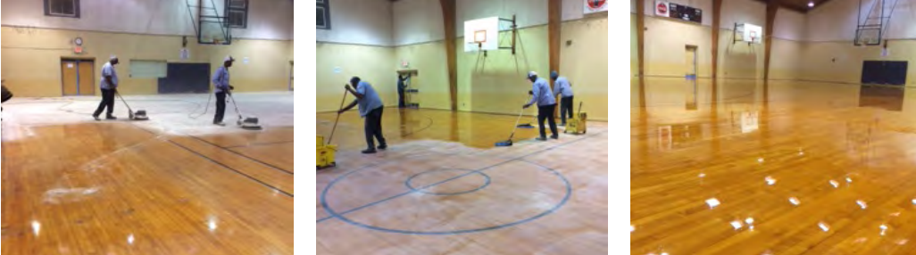
COVINGTON RECREATION CENTER — Willie Moss, Bobby Chambers and Elmer Norris sanding and refinishing the gymnasium floor in the Covington Recreation Center.
