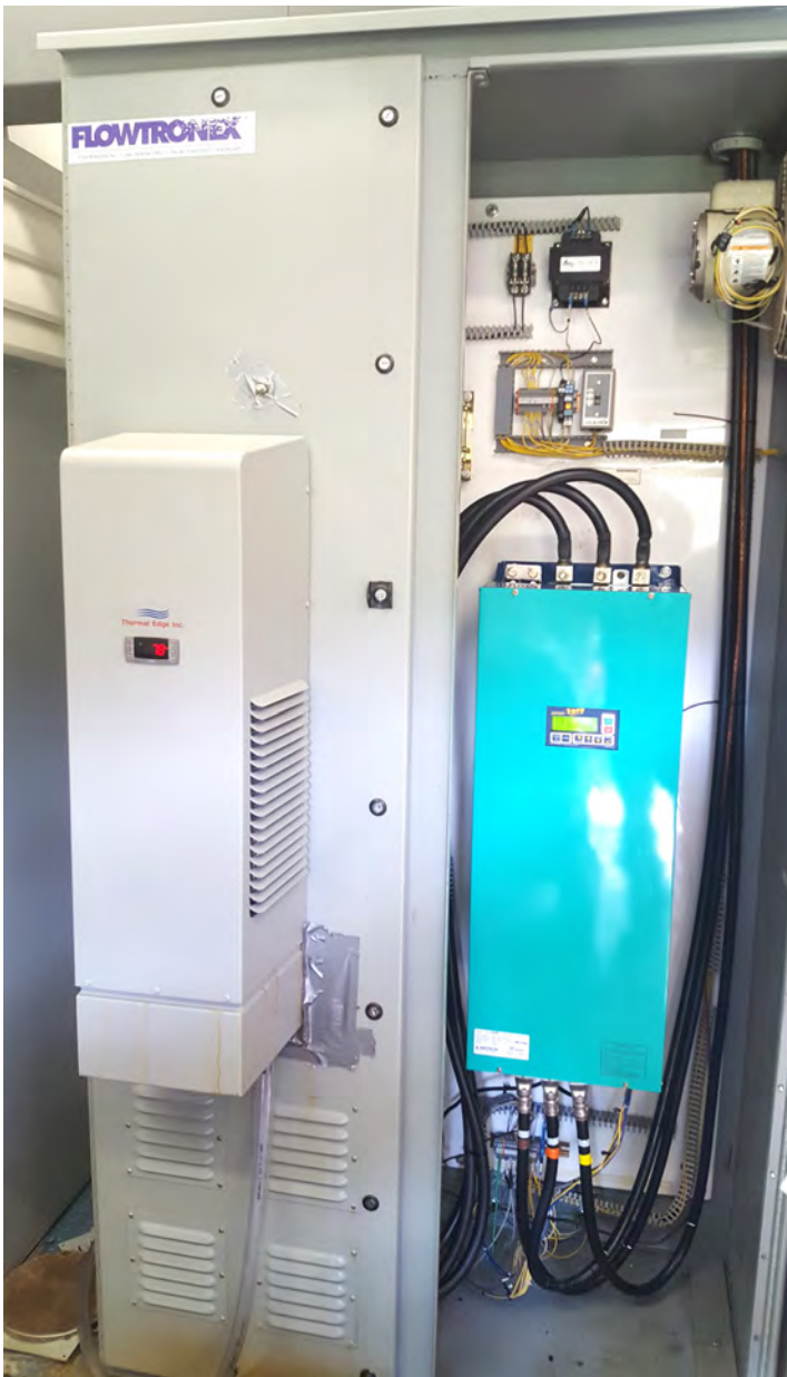
Forsyth County's Dicks Creek Drive
