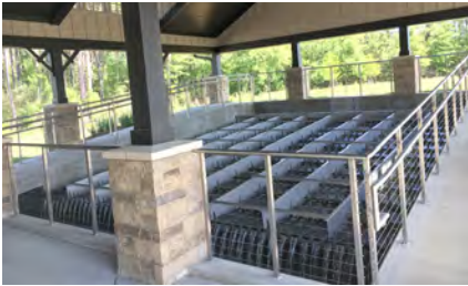
Cascade Aerator at New 6 MGD Wastewater Treatment Plant Administration Building
