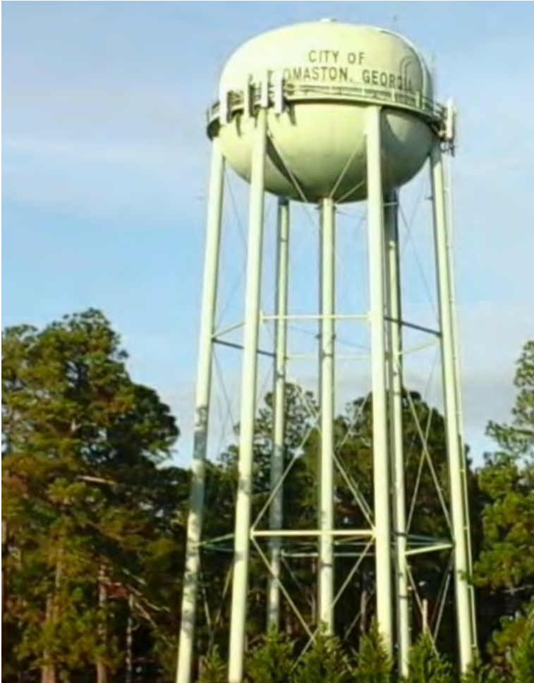
THOMASTON'S SILVER TOWN ELEVATED WATER STORAGE TANK
