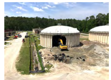
FORT STEWART WPCP ABANDONED TRICKLING FILTER DEMOLITION
