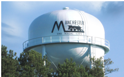
Macedonia Tank AFTER renovation
