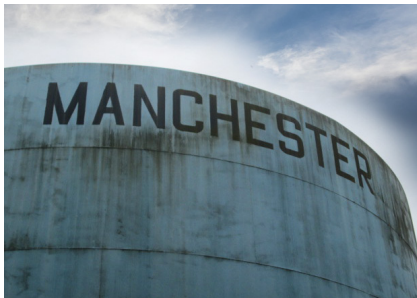
Mayes Way Tank BEFORE renovation
