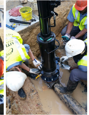
C&D Crew installing new valve
