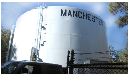
Mayes Way Tank AFTER renovation
