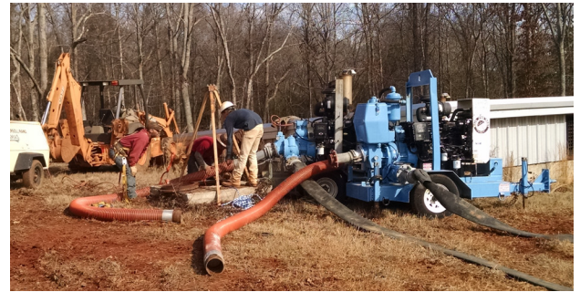
Bypass Pumping • Wastewater Treatment Plant
