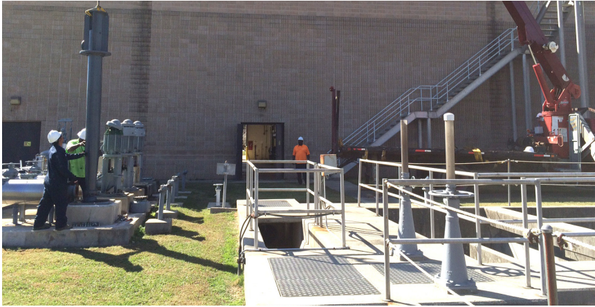
Reuse Pump Installation
