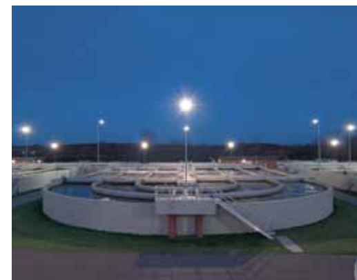
Photograph 1 (top) • Headworks Photograph 2 (bottom) • Basin #2
