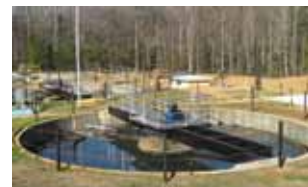
Left: Secondary Clarifiers before Right: Secondary Clarifiers after
