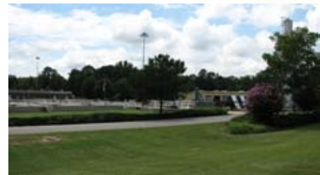
▪ Sandy Run Wastewater Treatment Facility
